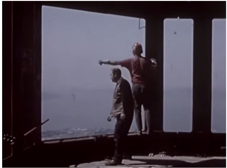
WTC construction, example of a corner hole, UAL175 engine exit ( Source )
